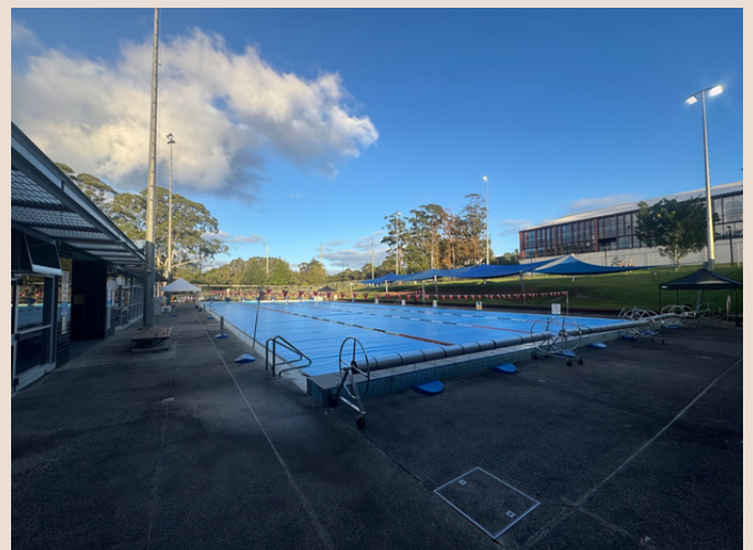
50m pool with change room access.
