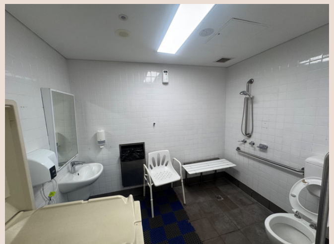
Inside accessible bathroom/family change room.
