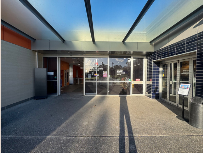
Automatic doors at entrance.
