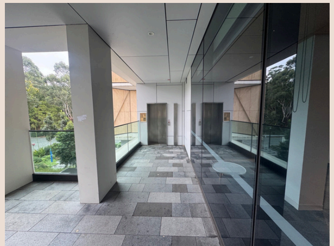
Lift/Elevator leading downstairs.
