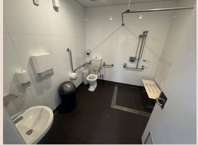
Accessible bathroom next to male and female change rooms. Level 1
